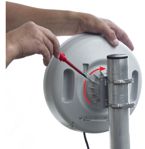
11 While holding the StationBox in desired position, tighten the Nut as much as you can. Optional: To secure the position, use Security Screw that cuts in the Ball part of the bracket.
